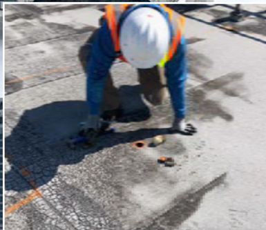
CORING THE ROOF - CHECKING FOR MOISTURE!
