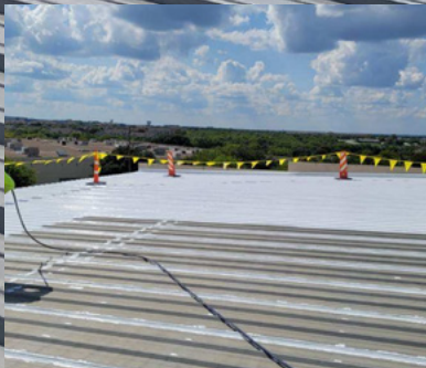
MAKING ROOFS WATER-TIGHT!
